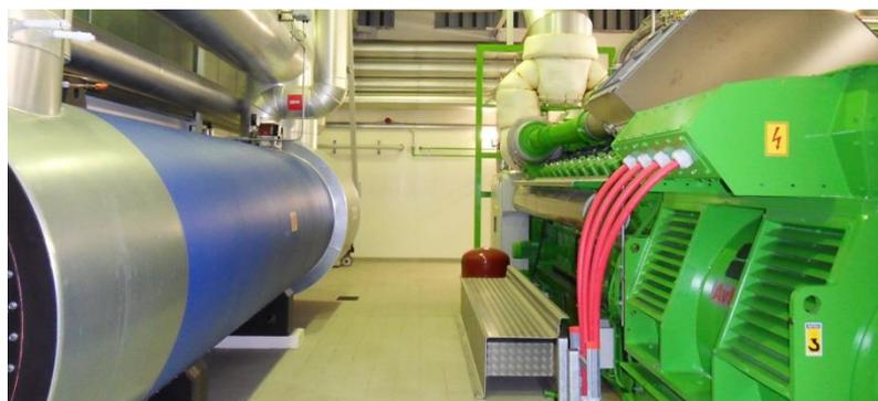
Figure 1: CHP Engine at TCMK energy centre.
